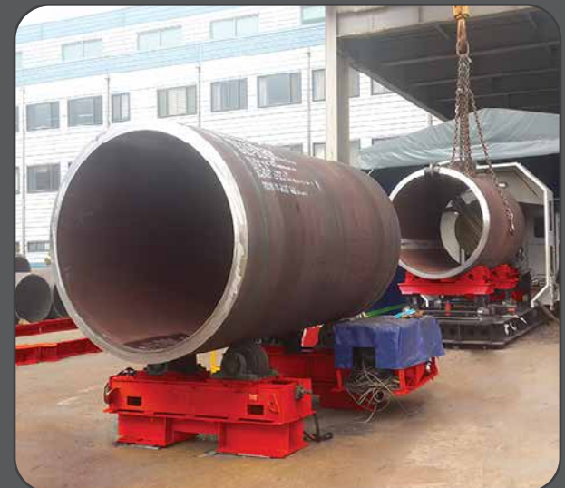
Giant Pipe Beveling
